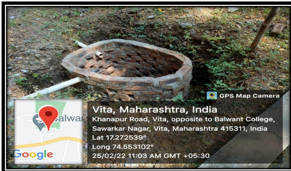
Hazardous Liquid Waste Soak Pit for Chemistry Laboratory
