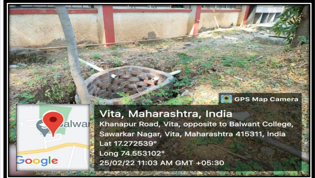
Liquid waste absorbing Soak Pits on the college campus.
